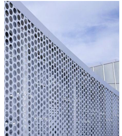
Fig.6.17 - Element's Geometry: Circular Elements - New Center for Manufacturing Innovation in Monterrey, Mexico (source: www.archilovers.com/ )
