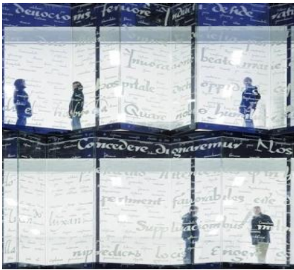
Fig.6.51 - Facade's Material: Glass - an example of a printed facade - Historical Archive of the Basque Country in Bilbao, Spain (source: www.archilovers.com/ )
