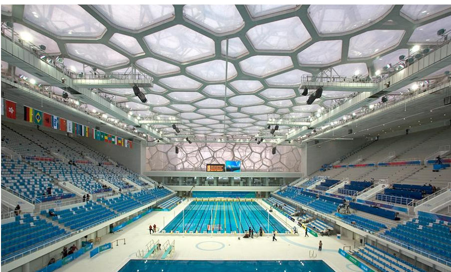
Fig.4.15 – Interior of the Water Cube pavilion (source: http://www.arup.com/Projects/ )
