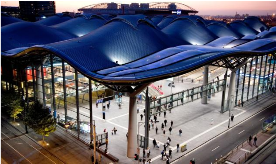
Fig.2.19 - Photography of Southern Cross Station in Melbourne, Australia (source: http://openbuildings.com )
