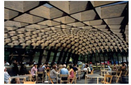
Fig.4.4 - Serpentine Gallery Pavilion 2005 by Alvaro Siza and Eduardo Souto de Moura with Cecil Balmond – Arup (source: http://www.telegraph.co.uk/ )
