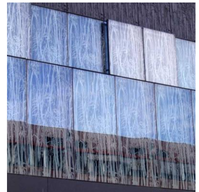
Fig.6.43 - Facade's Articulation: Printed Facade - Utrecht University Library in Netherlands (source: www.e-architect.co.uk/ )
