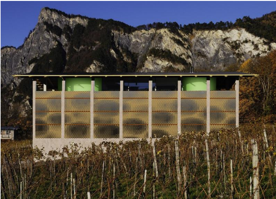
Fig.9.53 - The model of the Gantenbein Vineyard with a grid producing the facade pattern of the grapes.
