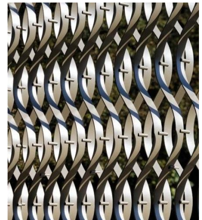
Fig.6.23 - Element's Deformation: Undulated Elements - Visitor Pavilion National Museum Palace in Het Loo, Apeldoorn, Netherlands (source: www.archilovers.com/ )
