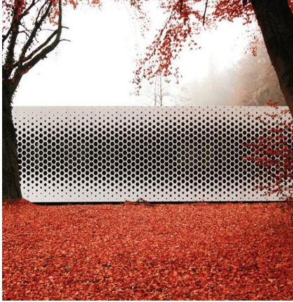
Fig.6.9 - Facade Geometry: Straight Facade - Formestelle Office Building in Töging am Inn, Germany (source: www.dezeen.com)
