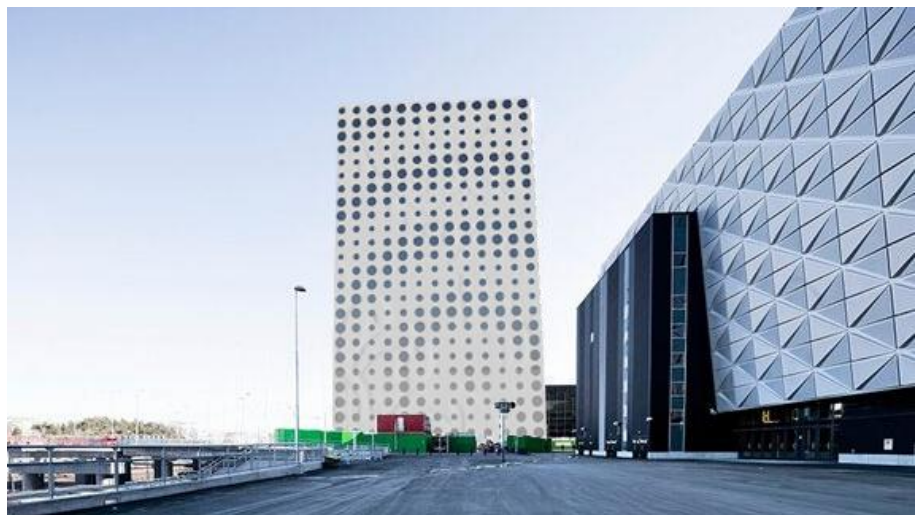
Fig.9.20 - An example of the Quality Hotel Friends facade produced by us: with 13X25 windows, the attractor point is (30 0 15) and the magnitude is 4.
