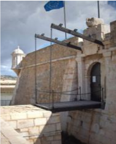
Fig.2.20 – An example of Kinetic architecture of the past: Drawbridge at the fort of Ponta da Bandeira in Lagos, Portugal (source: http://en.wikipedia.org/wiki/Drawbridge )
