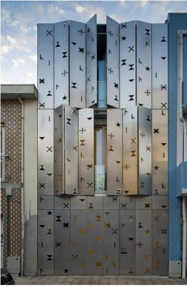
Fig.6.41 - Facade's Articulation: Perforated Facade - House 77 by Diniso Lab in Póvoa do Varzim, Portugal (source: www.dezeen.com/ )
