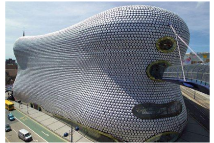
Fig.6.4 - Selfridges Building in Birmingham, UK (source: http://www.contemporist.com/ )
