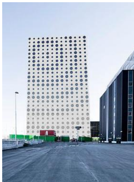
Fig.9.19 - An example of the Quality Hotel Friends facade produced by us: with 13X25 windows, the attractor point is (15 0 60) and the magnitude is 5.
