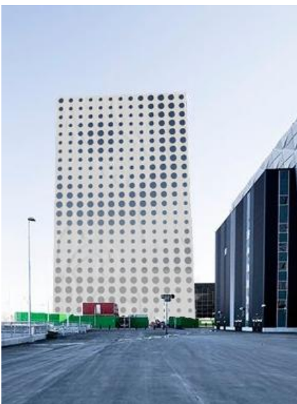
Fig.9.18 - An example of the Quality Hotel Friends facade produced by us: with 13X25 windows, the attractor point is (15 0 60) and the magnitude is 2.
