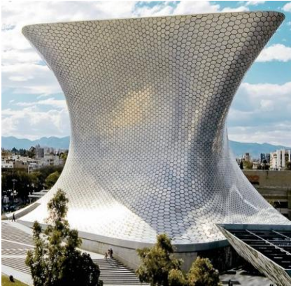
Fig.6.50 - Facade's Material: Metal - an example of a facade with a complex geometry - Soumaya Museum in Mexico City (source: http://www.archilovers.com/ )
