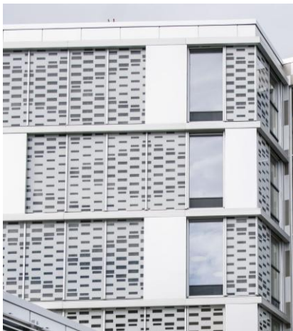
Fig.6.34 - Element's Distribution: in Chess-Grid - Knowledge center at St. Olav's Hospital, Norway (source: http://www.archdaily.com/ )
