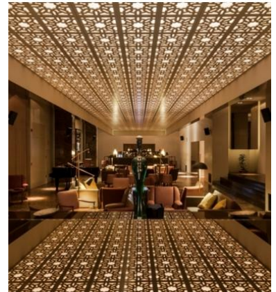
Fig.10.1 – False Ceiling: Bar Bô Zen in Braga by Central Arquitetos (source: http://centralarquitectos.com/ )
