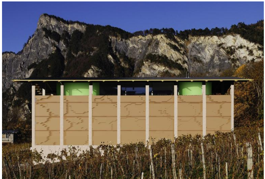
Fig.9.47 - The model of the Gantenbein Vineyard with bricks placed backward and forward.
