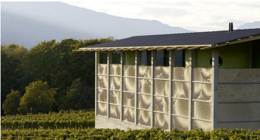
Fig.6.40 - Element's Rotation: Pictorial Rotation - Winery Gantenbein by Gramazio & Kohler, in Switzerland (source: http://www.gramaziokohler.com/ )
