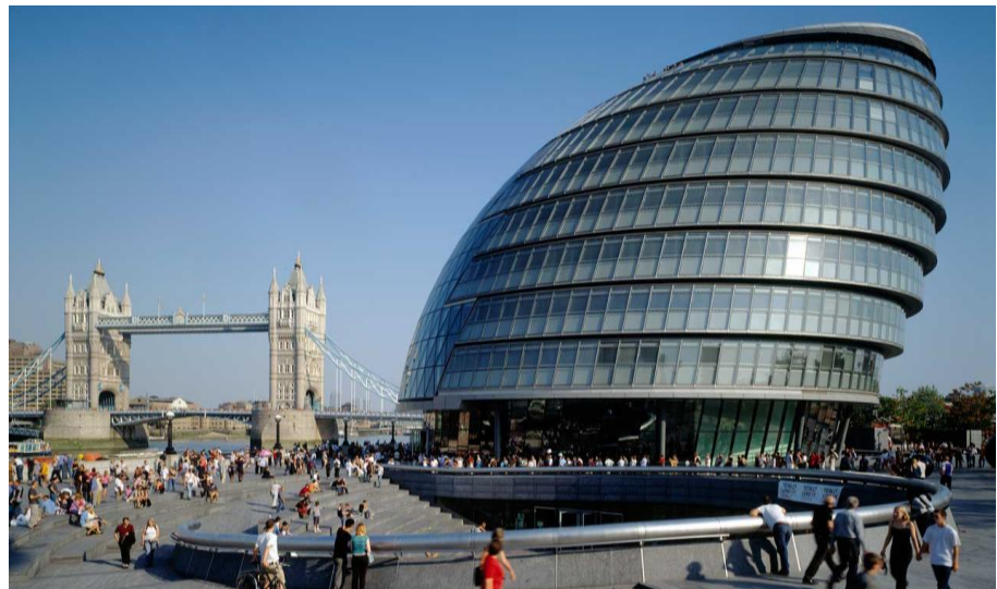
Fig.2.16 - Photography of the City Hall in London, designed by Foster+Partners (source: http://www.fosterandpartners.com )
