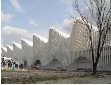
Fig.6.14 – Facade’s Geometry: Facade with vertical and horizontal waving - Mediopadana Station in Bologna, Italy (source: www.ediliziaeterritorio.ilssole24ore.com/ )
