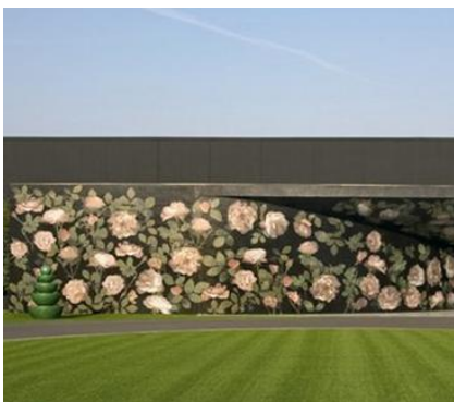
Fig.6.52 - Facade's Colors: Pictorial Color - The Bisazza Foundation in Alte di Montecchio Maggiore, Italy (source: www.archilovers.com/ )
