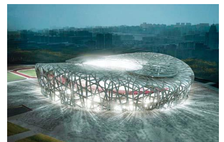
Fig.2.3 - A digital image of the Beijing National Stadium project by Herzog & De Meuron (source: www.openbuildings.com )
