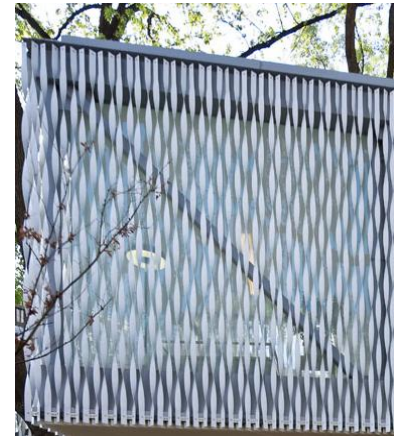
Fig.6.22 - Element's Deformation: Twisted Elements: Huaxin Business Center in Xuhui, China (source: http://openbuildings.com/ )
